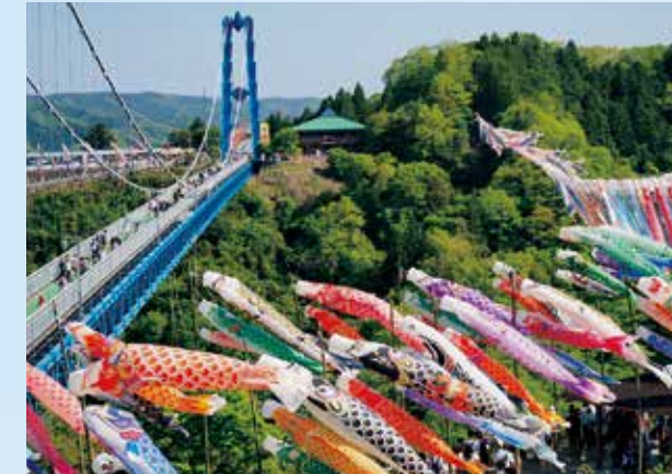
4 Ryujin Big Suspension Bridge
